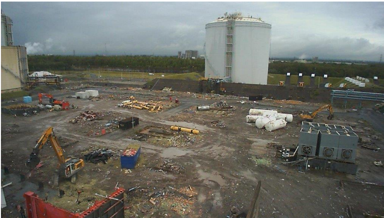
Partington during demolition
