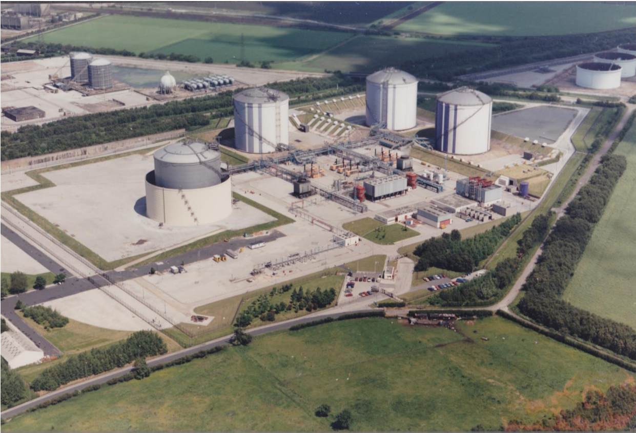
The Partington site showing the four LNG storage tanks in the mid-1980s
